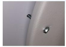
**PROBLEM:** Ceiling cobbled together with makeshift pieces visible from the OR. **CAUSE:** Installers "just making it work."
