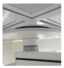
**PROBLEM:** Boom overlap on framing leaves large gap for contaminants to leak into room from above the ceiling. Unprofessional appearance.
