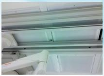
**PROBLEM:** Medical equipment obscuring diffusers. Filter access requires disassembly of all attached equipment.
